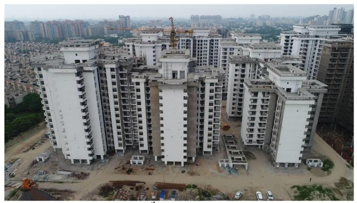
In Block B-03 11<sup>th</sup> floor Roof slab 75% casted. 12<sup>th</sup> floor columns casting is in progress.
